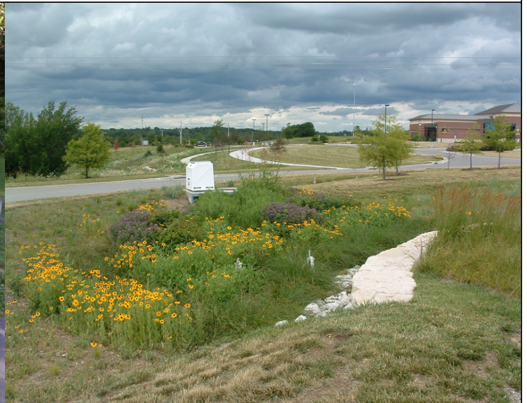
Photo 2. Typical bioretention basin
