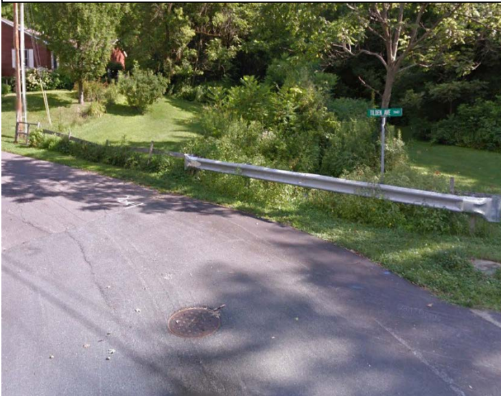
Photo 1. Corner of Millet Street and Tilden Avenue where stormwater enters the closed drainage system
