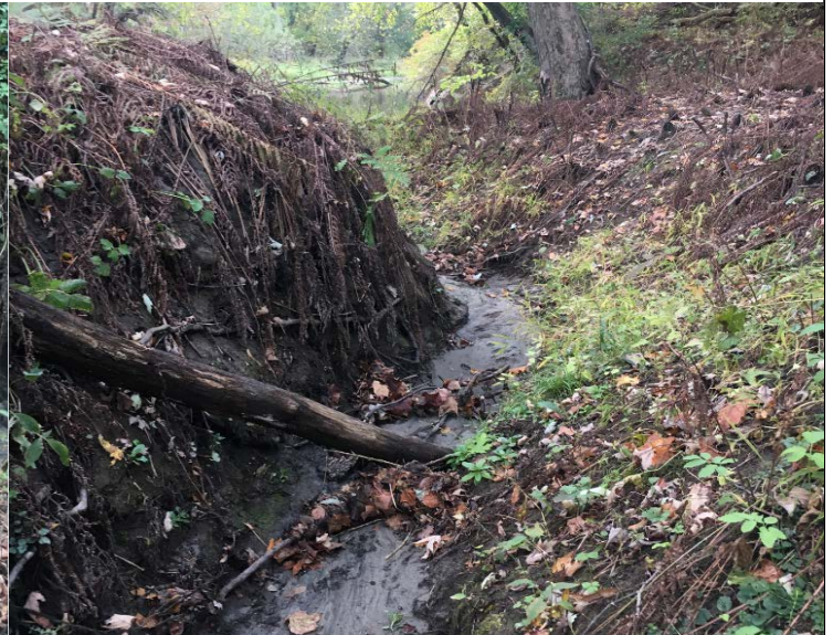
Photo 2. Eroding drainage ditch and its junction with the pond
