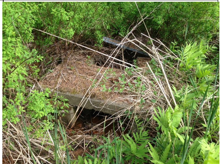
Photo 2. Existing inlet structure for the culverts passing beneath I-89.
