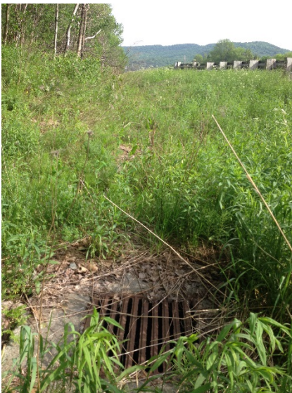
Photo 1. Potential BMP area, looking south.
