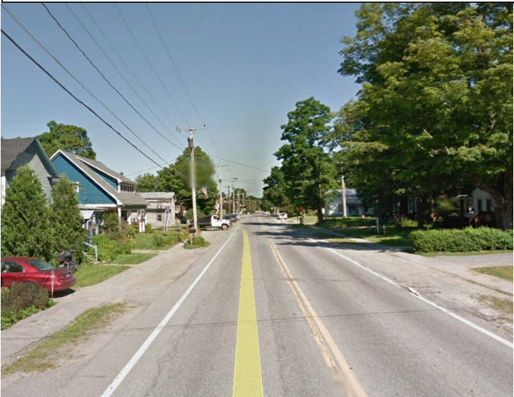
Photo 1. Main Street looking west depicting deteriorating green strips and sidewalks that could be used for stormwater treatment.
