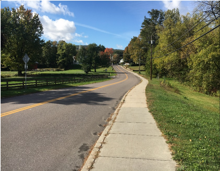
Photo 1. Portion of the WR-03 drainage area
